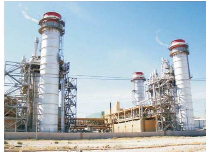
SAMRA power plant expansion project unit engineering in Jordan
