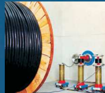
HV Partial Discharge Room
