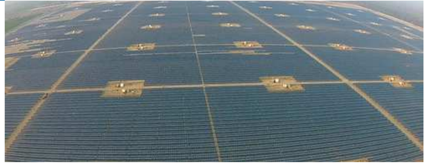
100 MW solar photovoltaic power generation project in Abubakar Jinnah solar Park in Pakistan
