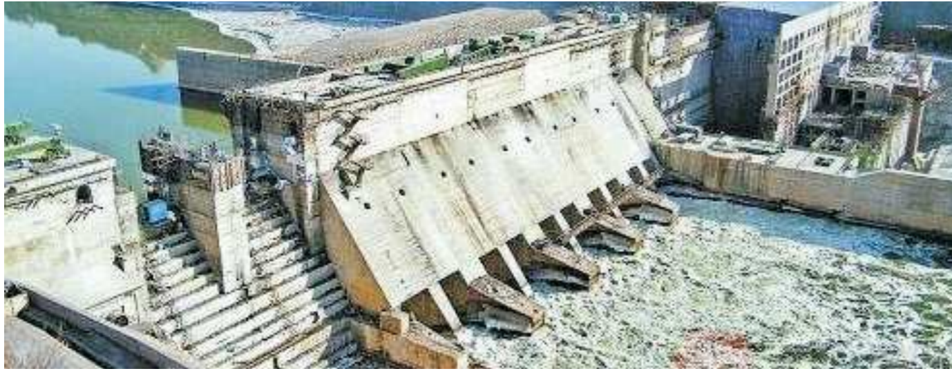
Karuma hydro power station and transmission and transformation project in Uganda
